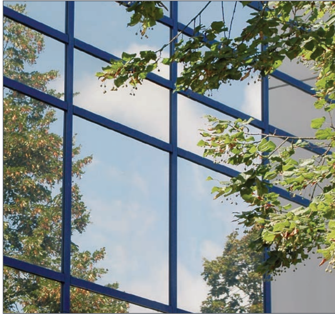
Glass with high coefficient of reflection
